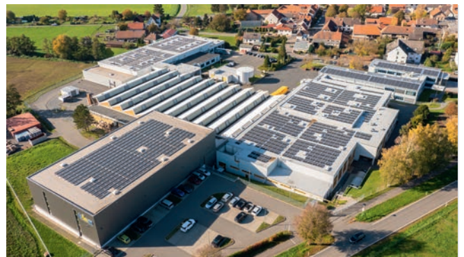
With social responsibility and photovoltaics on the roofs: the company headquarters is located in Ober-Ramstadt in the south of Hesse.
